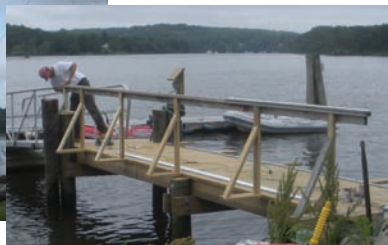
New pilings and dolphins were installed at the north and middle docks along with a much improved ramp.
