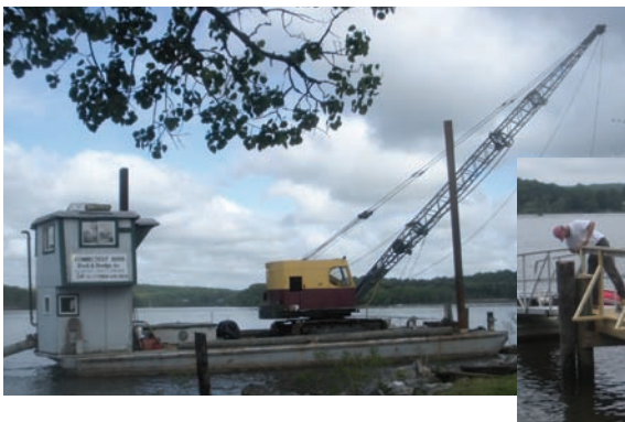
New pilings and dolphins were installed at the north and middle docks along with a much improved ramp.
